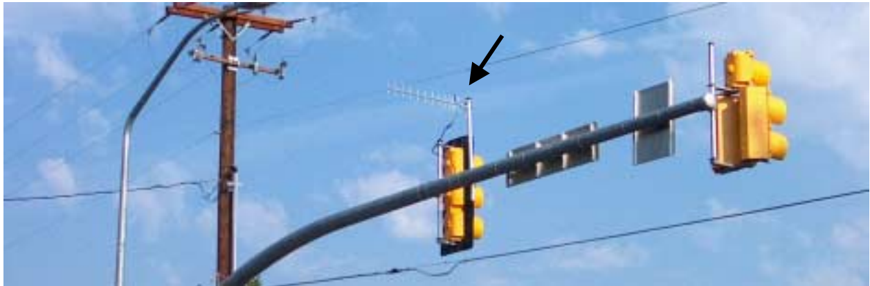
Exhibit 3.1 - Directional Spread Spectrum Antenna
